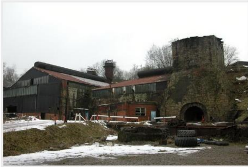
Photo 1: General view of Steelworks site with Blast Furnace No . 1 (right) and Wilkinson Foundry (middle with extension to the left).
