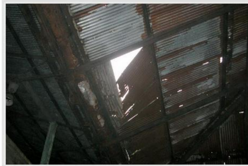
Photo 5: Condition of Foundry roof structure.
