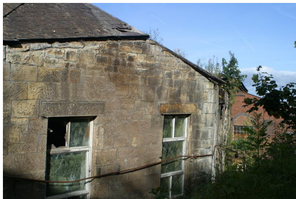
Rear view of Pattern Makers Shop
