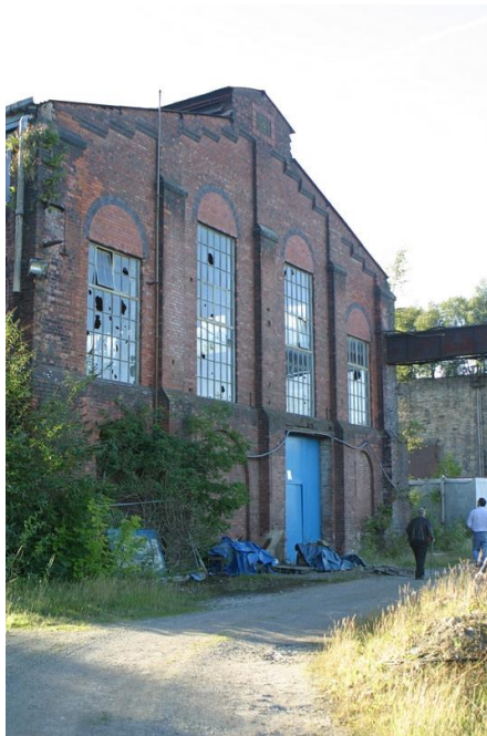
Rear of Machine Shop
