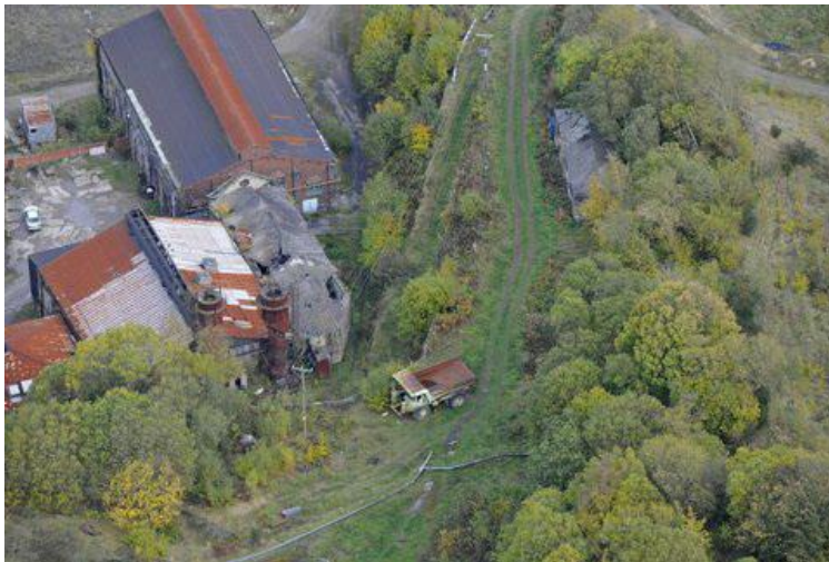
Key structures (note the condition of the Pattern Makers Shop : Agents House is seen to the right)
