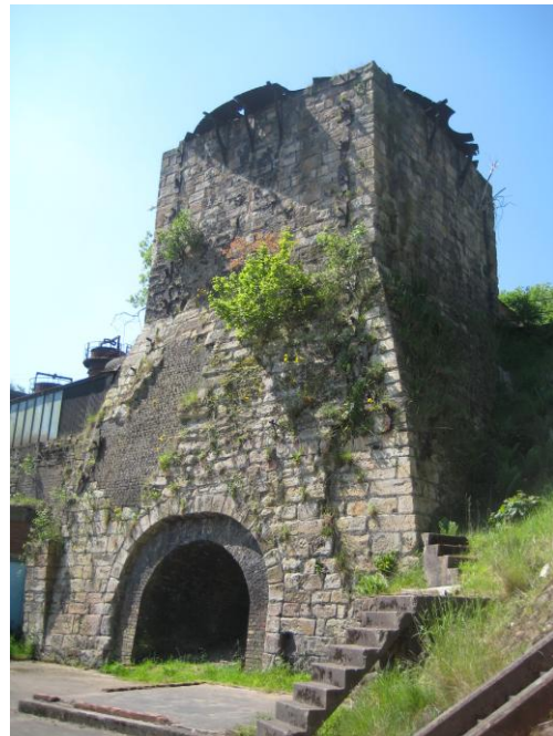
No. 1 Blast Furnace
