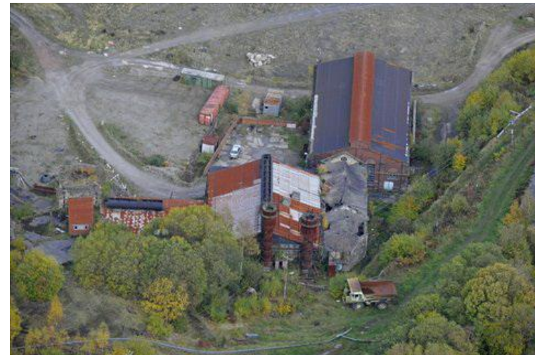
Key buildings of the Heritage Area (No. 1 Blast Furnace, Foundry and Pattern Maker's Shop are an integrated group below the Machine Shop)
