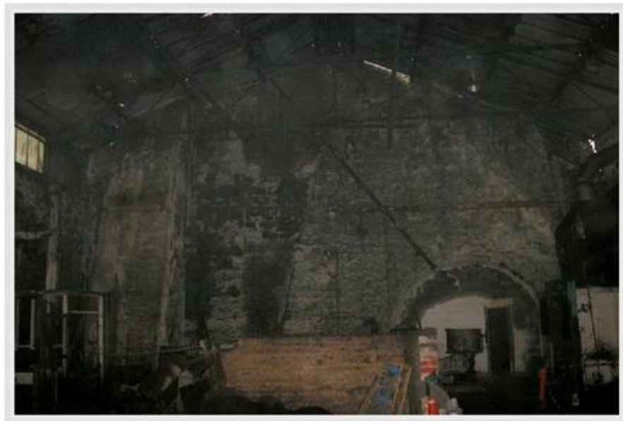
Photo 4: Interior of Wilkinson Foundry.
