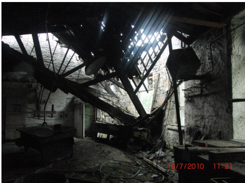
Current condition of the Pattern Maker's Shop
